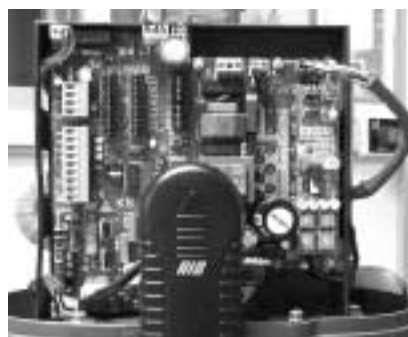
Final view of the assembly.
